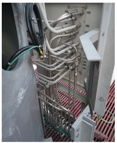
*Figure: Photo taken during site survey of the tubes that required isolation valves.*
